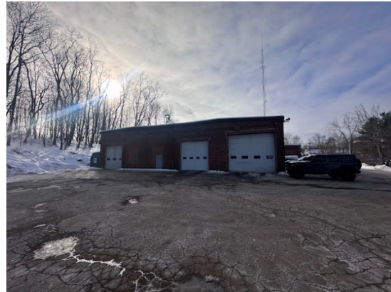
Existing Merrimac DPW Building & Yard 16 East Main Street
