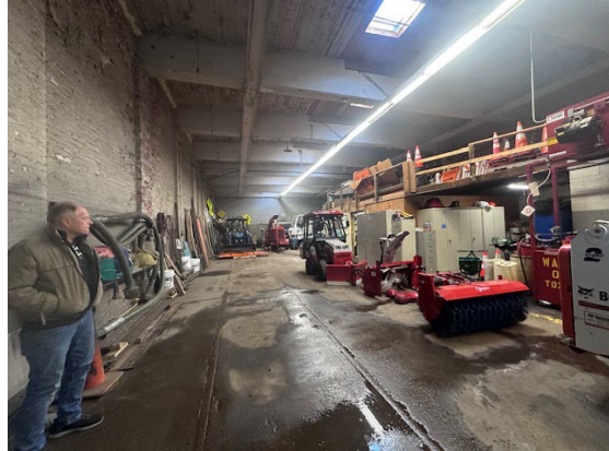
Existing Merrimac DPW Maintenance Bay
