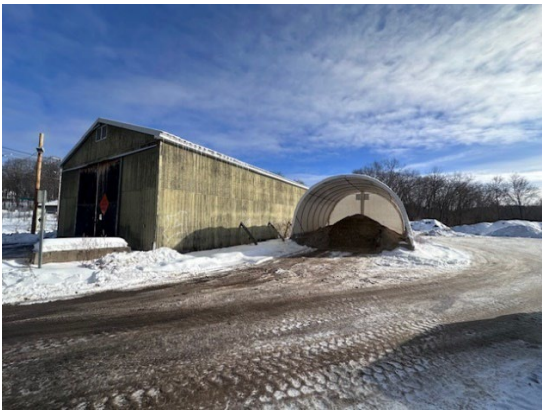
Federal Way Salt Storage
