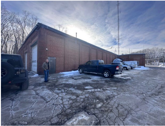
Existing Merrimac DPW Building 16 East Main Street
